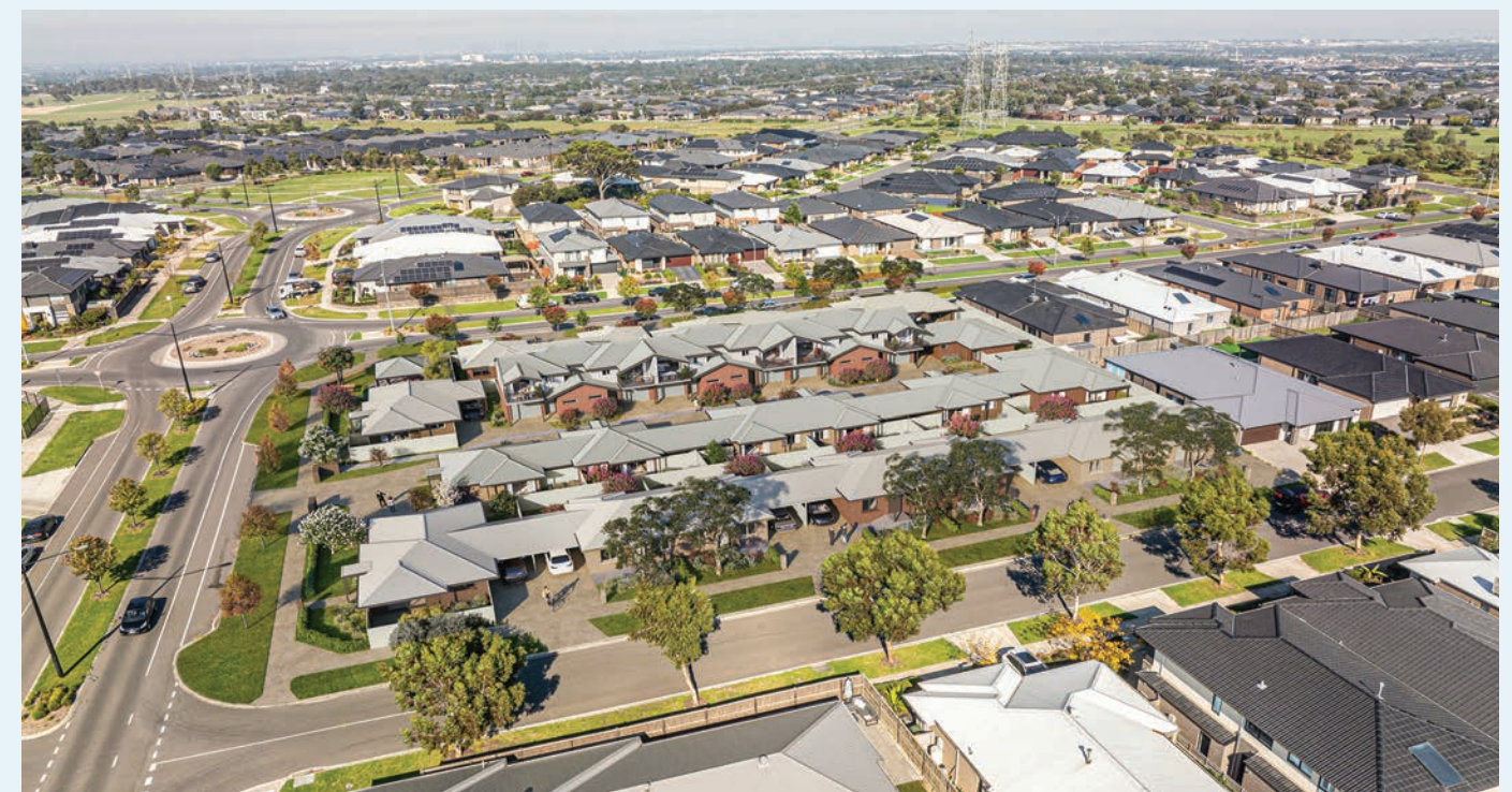
Aerial image showing the overall layout of the development.
