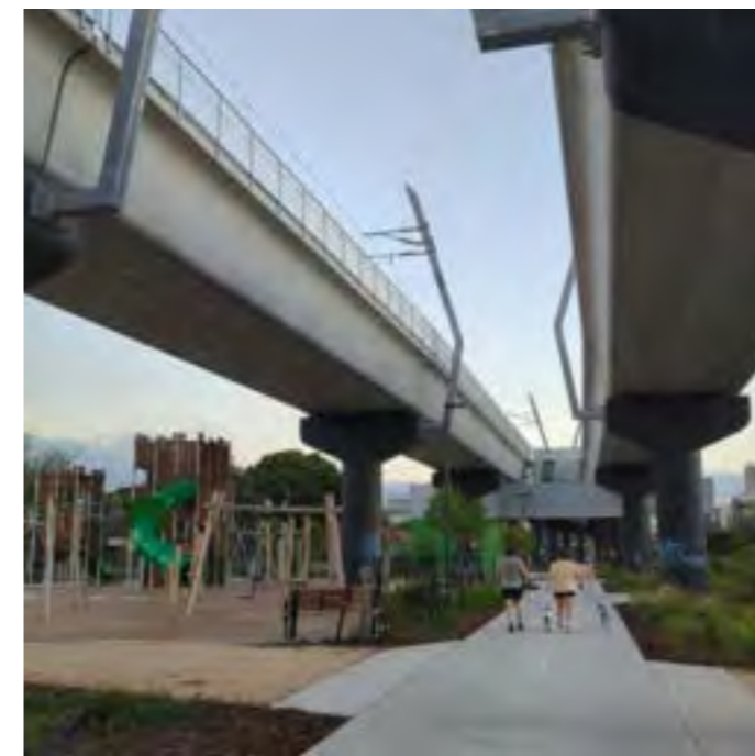
Figure 26 Linear park playground under elevated rail corridor between Bell and Preston station
