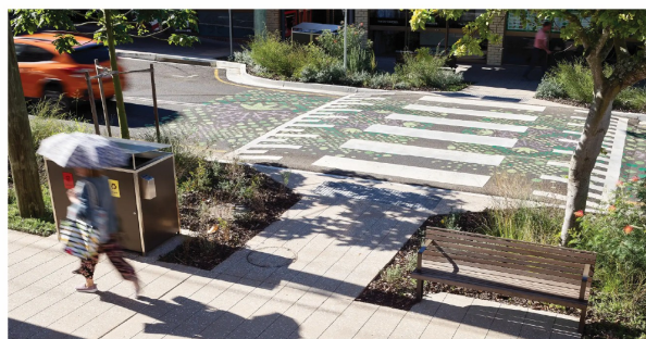
RAISED PEDESTRIAN CROSSINGS
