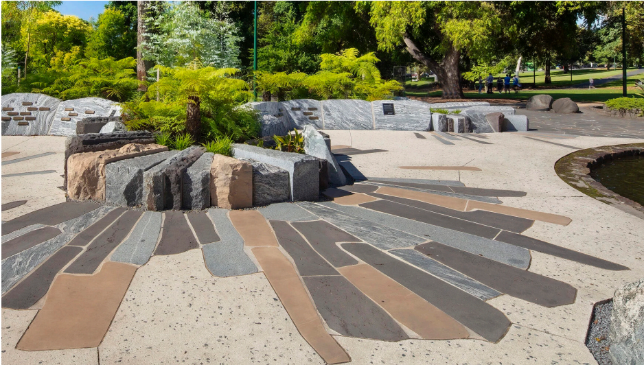
2. STONE PAVING INLAY TO CONCRETE PATH
